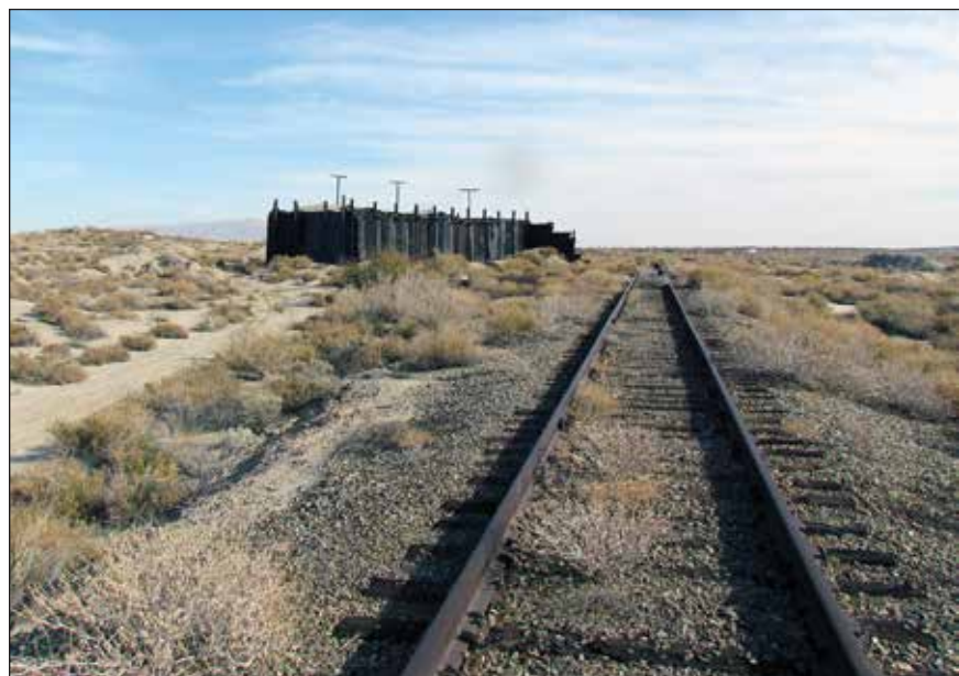
Ferrum Junction and maintenance building.
