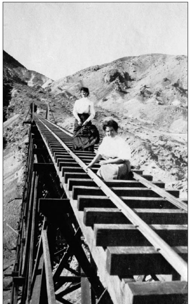
Figure 2. These two dare devils pose on the newly completed trestle
