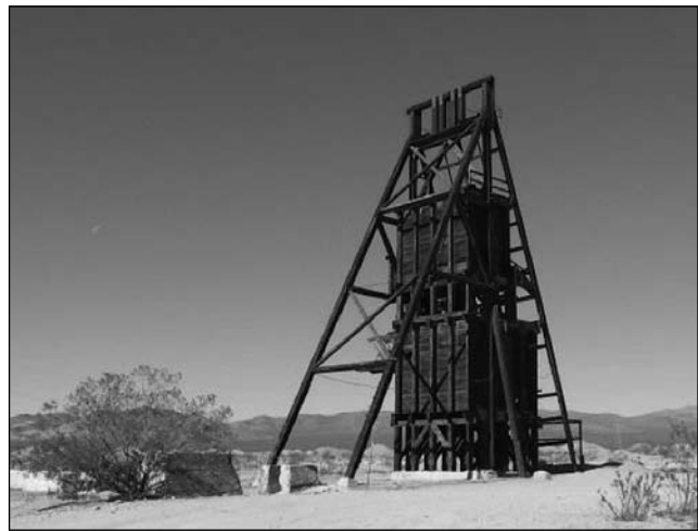
Figure 1-1. Union Tungsten Mine headframe. [J. Westbrook photo]
