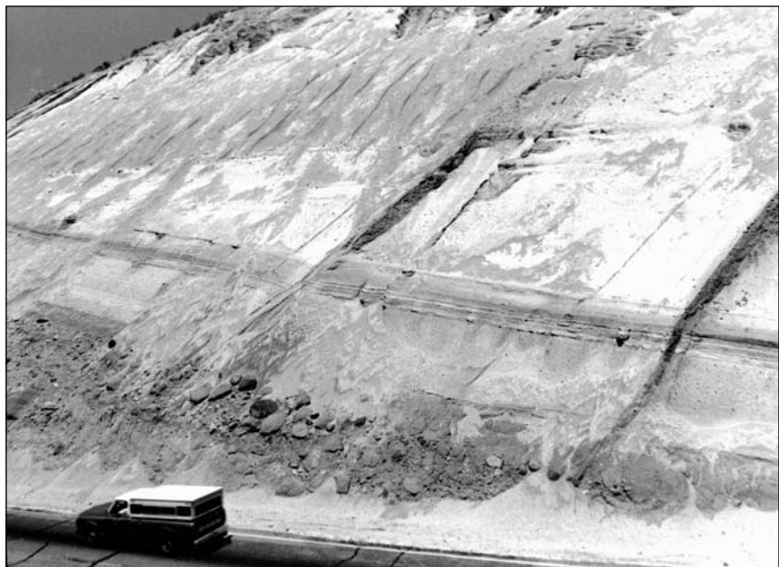
Figure 2-5. The “Big Pumice Cut” along Highway 395. The bouldery Sherwin Till is overlain by Bishop Tuff. The basal air-fall tuff is overlain by a much thicker ash-flow. An angular unconformity separates the units. Several prominent “clastic dikes” cut the tuff layers. [Photo by S. Lipshie, 1976]
