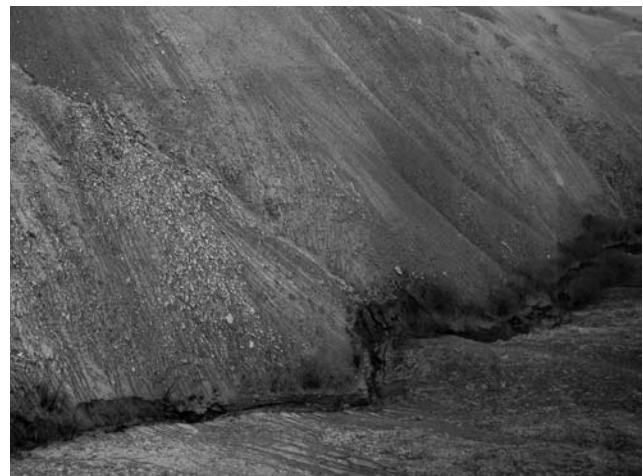
Photo 7. Rilling of slopes in Charlie Canyon. Photo by Jerry DeGraff.
