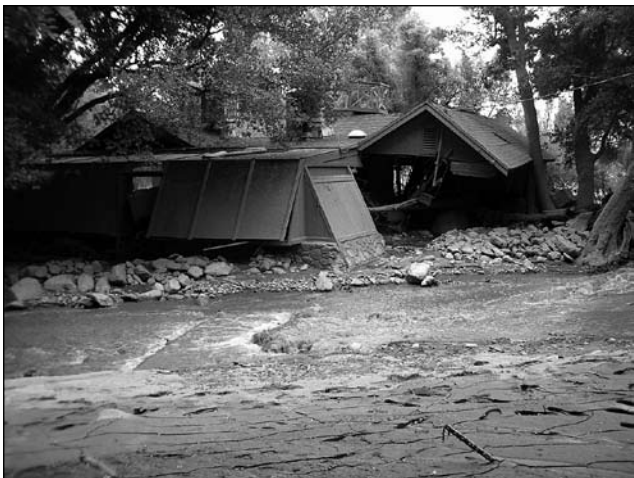
Photo 14. This house took a direct hit by mud and rocks. Note large boulders and tree visible in interior. Flow went in the west side and out the east. View south. Creek on north side of house after partial realignment, but not in original channel. Photo by Jim Stroh.
