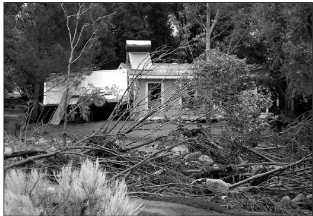
Photo 13. Double-wide mobile home moved to the right (east) off its foundation and rammed into trees. Trailer was salvaged. Photo by Jim Stroh.
