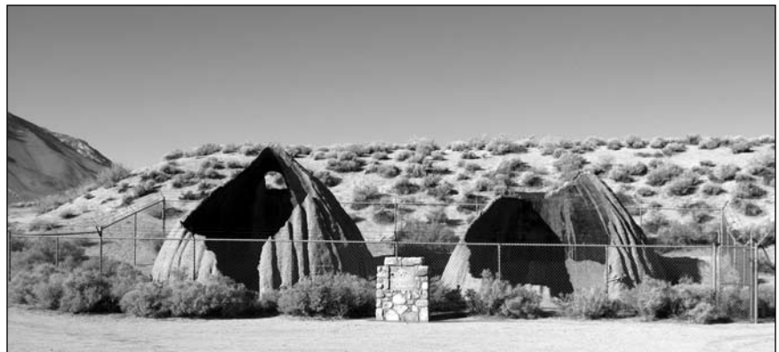
Figure 1-8. Stop 1-4. The Cottonwood charcoal kilns. [Reynolds photo]
