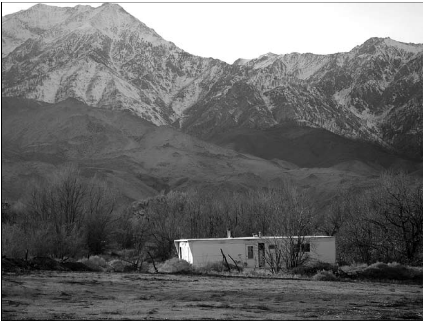
Figure 3-2. Mobile home damaged by the Oak Creek debris flow. [Reynolds photo]
