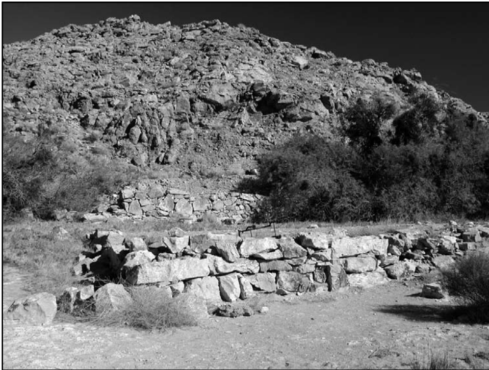
Figure 4. Dry-laid retaining walls forming building pads (?) near the foundations in figure 3. R. Fulton, photo.
