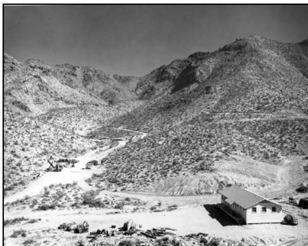
Bunkhouses and mess hall, looking northwest toward the orebody. Photograph from the Bud Davenport collection, Mojave National Preserve.
