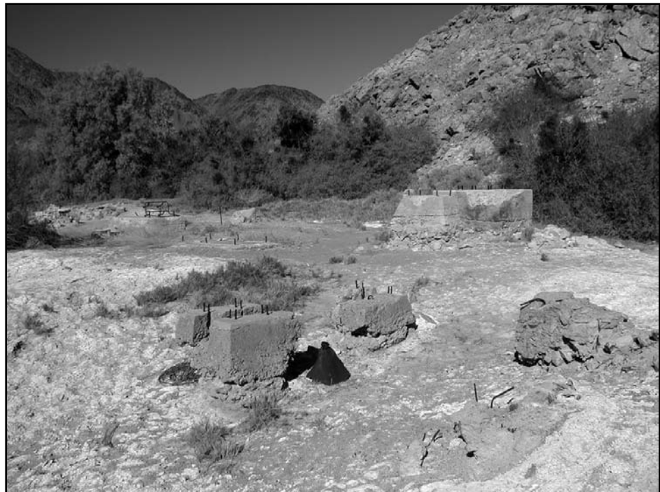
Figure 3. Concrete equipment foundations (?) of the Pacific Coast Soda Co. at the south end of the limestone ridge, just west of ponds seen in figure 2. R. Fulton, photo.
