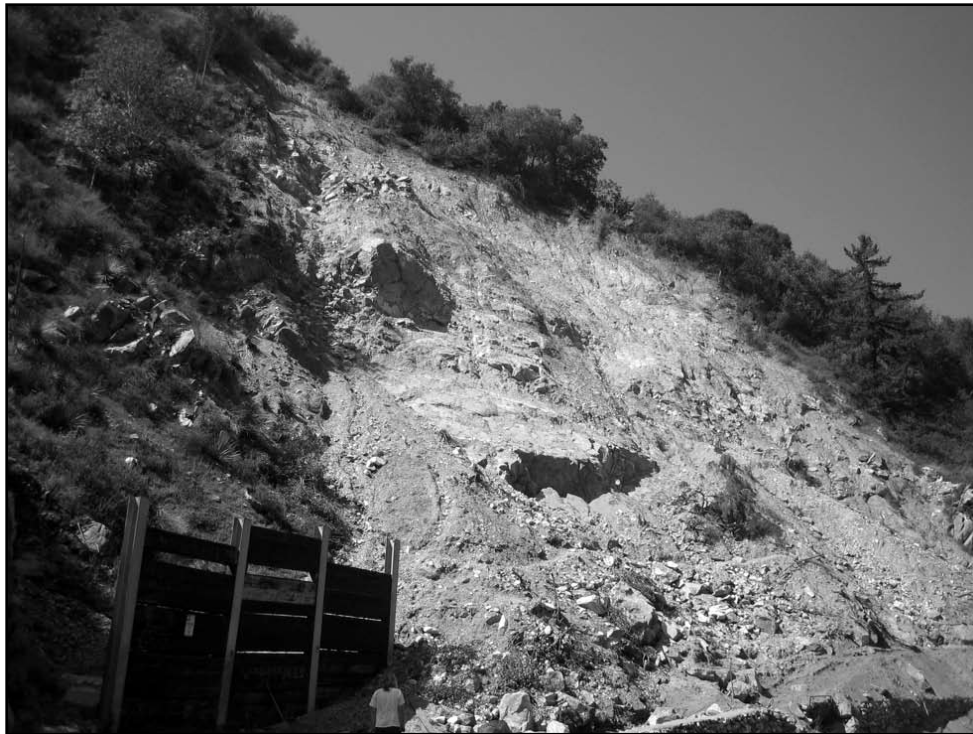
Figure 4. The Pine Slide looking northwest.
