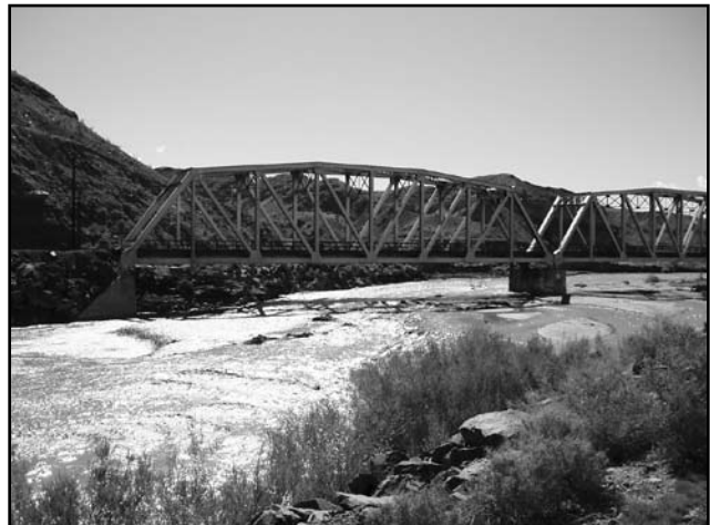
East Afton trestle.
