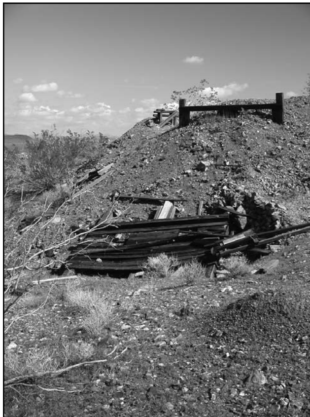
Loading bin at the Gold Hammer Mine. R.E. Reynolds photograph.
