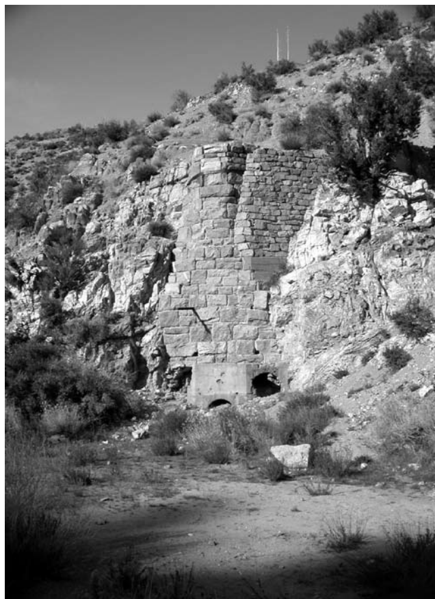
PHOTO 3-1, STOP 3-4. View north of a lime kiln built with blocks of angular local rock.
