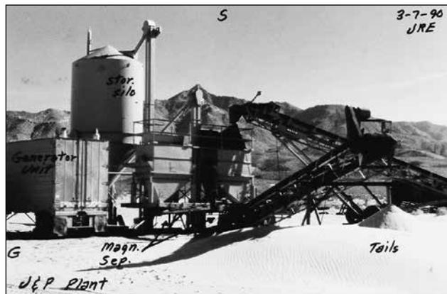
J.P. Project processing plant, showing conveyors, magnetic separation unit, and magnetic concentrate storage silo and generator unit. Photo taken 3/7/1990 by J.R. Evans.
